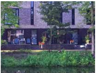
In 't Zuiderpark Fase 1 - Inbo Rotterdam, Netherlands
